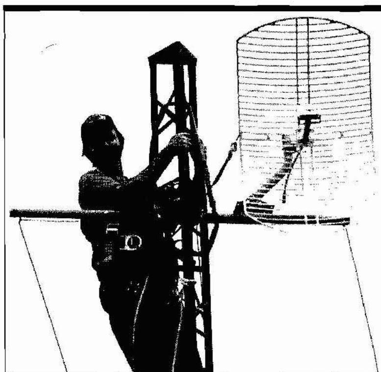
Daryl, KG4PRR, installs a microwave reflector array.
